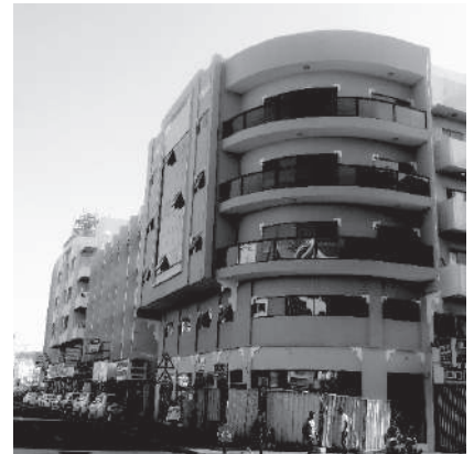
Al Rams Building, Dubai
