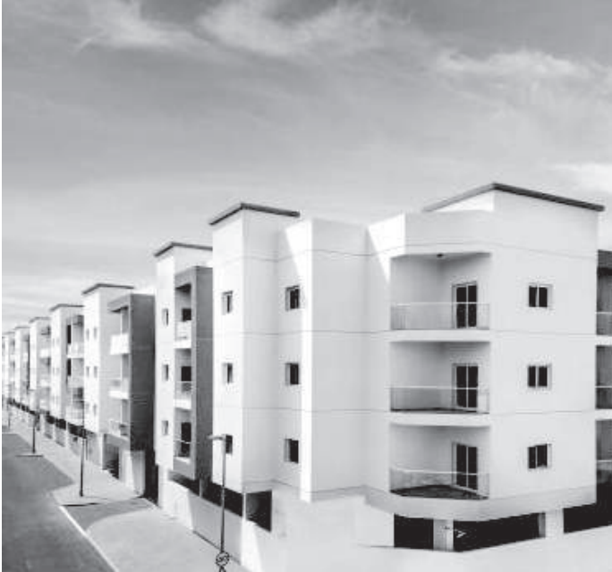
EOL Works of Flats, Idama, Al Wasl Properties
