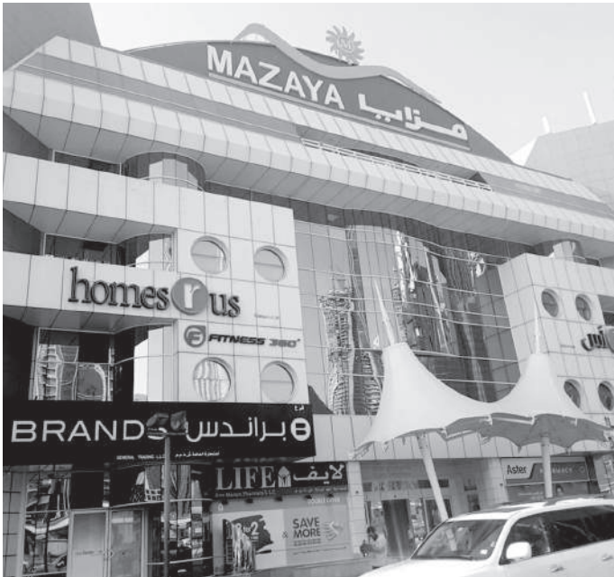
Rooftop Waterproofing and GI Cladding Works, Mazaya Center, Wasl Properties
