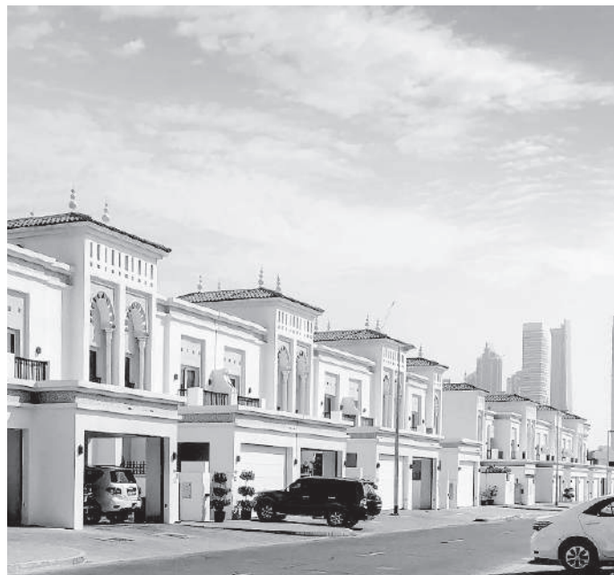
EOL Works of Villas, BK Gulf, Al Wasl Properties
